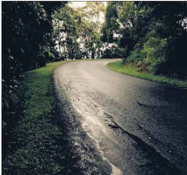
Federal resident Brad Garnham says this corner on Coolamon Scenic Drive needs urgent repair. Photo supplied
