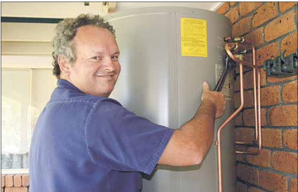
Gasfitter Peter Thompson adjusts plumbing on a new 400-litre hot-water tank at Nunderi heated by a solar heat pump. Rebates are available to residents installing solar hot-water systems, rainwater tanks, insulation or even washing machines.
