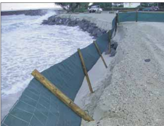
Tidal erosion in the past week has again played havoc with the Kingscliff Beach foreshore and battered a recently-installed safety barrier. Photo Chantal Bradshaw
