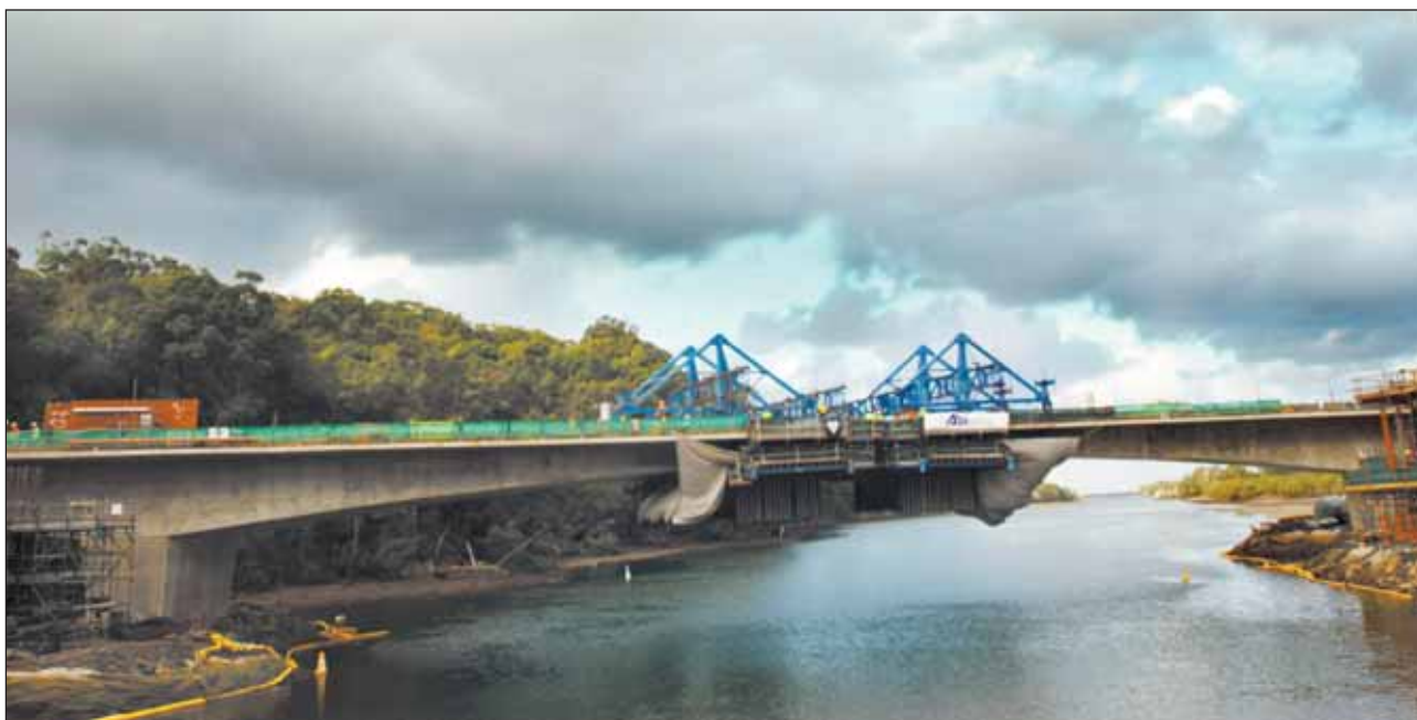
Only about six metres now separates the north and south arms of the new bridge spanning the Brunswick River, although temporary formwork gives the impression that the two sections now meet. Over the next few weeks the gap will gradually close leaving the 180 metre span complete. Designed for eventual use by local traffic from Ocean Shores to Brunswick Heads, Pacific Highway traffic will be temporarily diverted from the existing roadway onto the ten metre high bridge by October or November this year to allow construction of a third bridge. Photo Jeff 'Bridge Over the River Why?' Dawson
