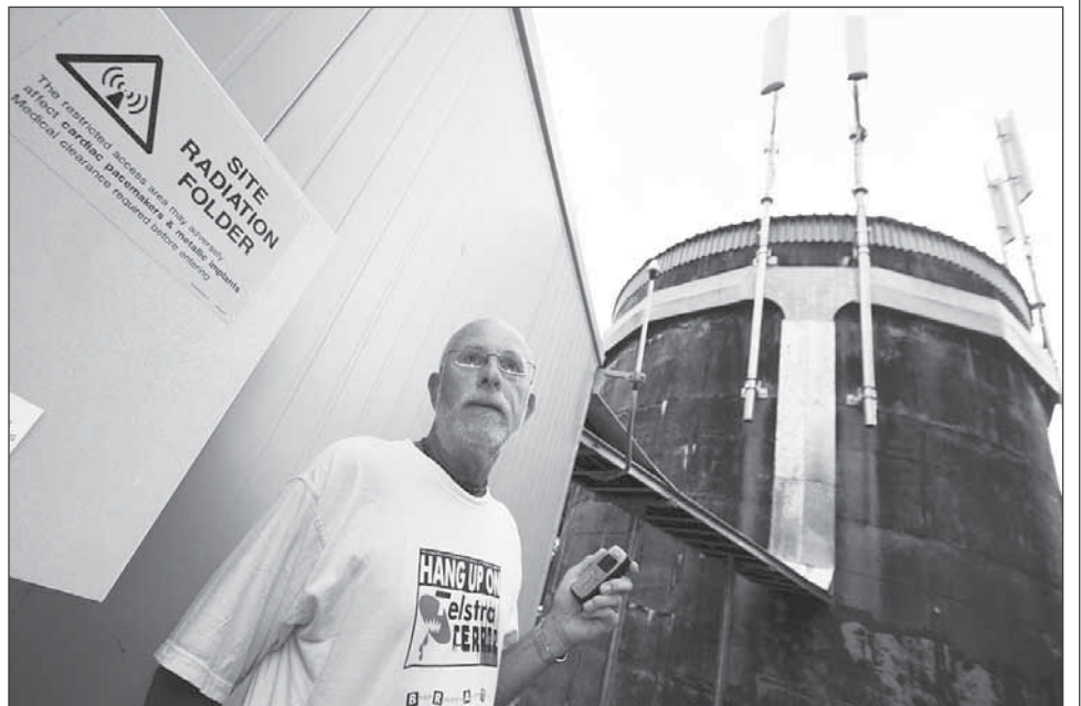
Peter Wegner next to the Suffolk Park water (and mobile phone) tower. Photo Jeff 'Cable Guy' Dawson
