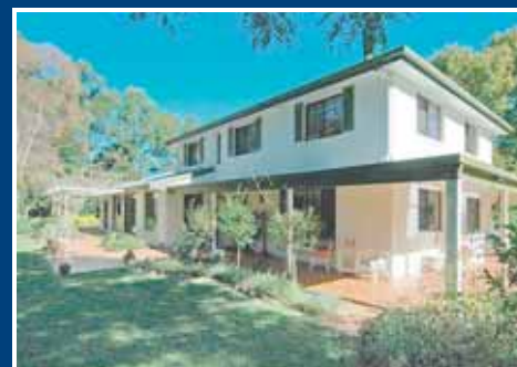
Gracious semi-rural manor $1,195,000 Semi rural, 7 bed/3 baths + media room 6473sqm of manicured gardens
