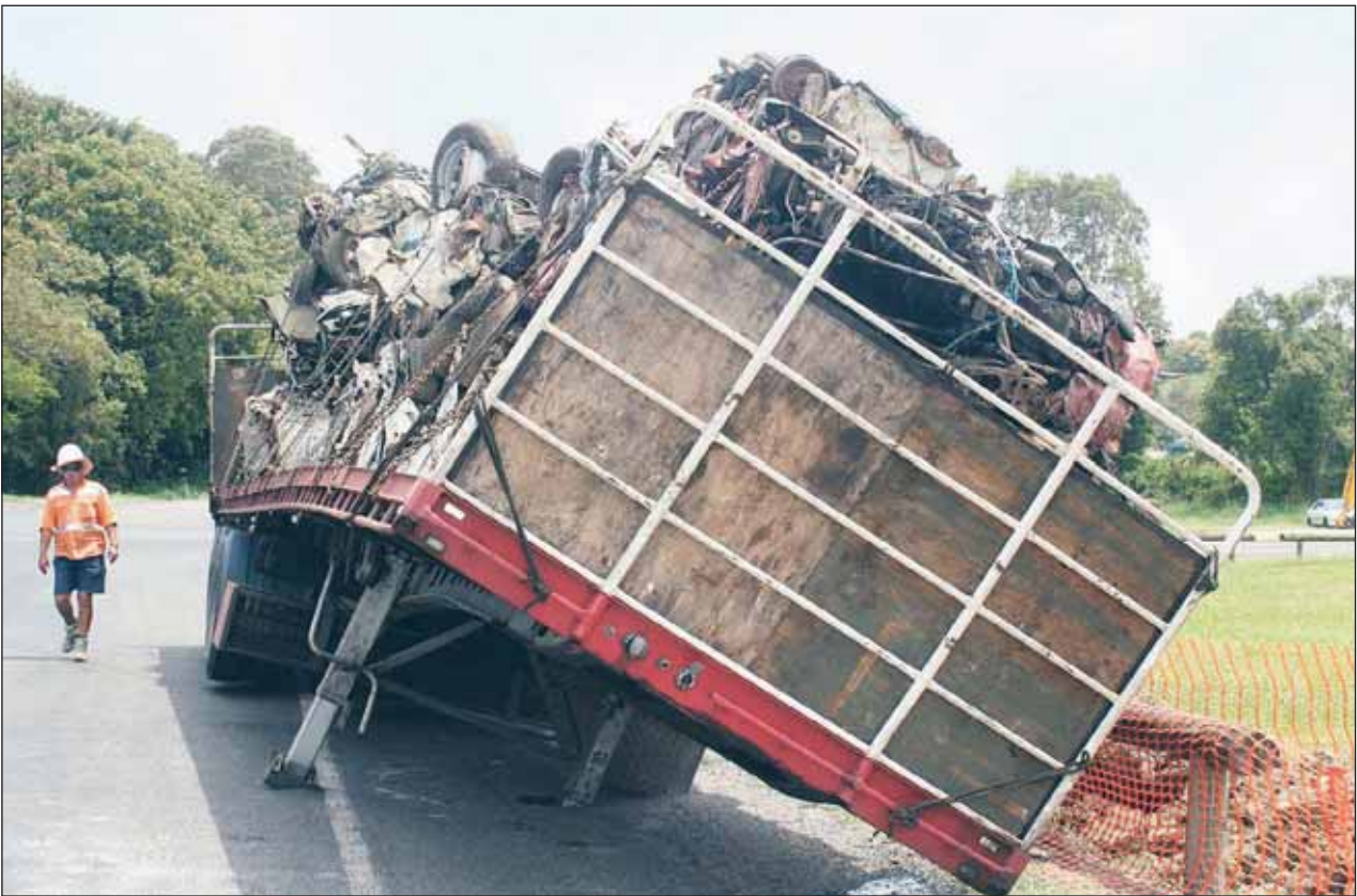
An unfortunate truck driver set up his rig at the Uncle Tom's turnoff only to discover it disappearing through the bitumen. Could it have anything to do with the hole Council workers were digging nearby? Photo Eve Jeffery
