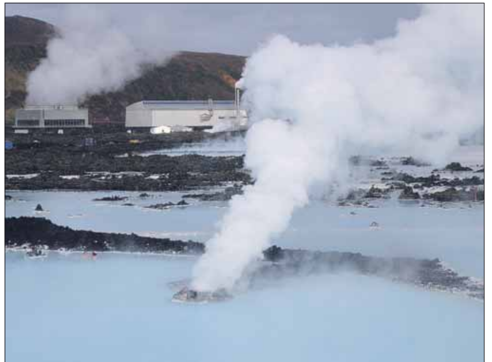
Geothermal facilities near Grindavik, Iceland. From Wikimedia Commons.
