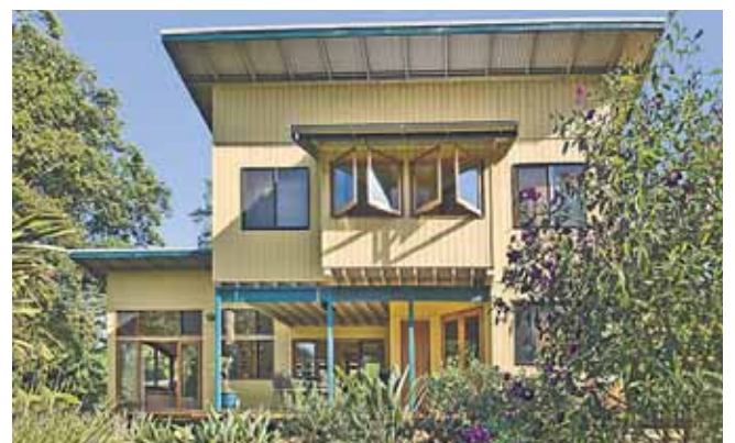
511 Friday Hut Road, Possum Creek
