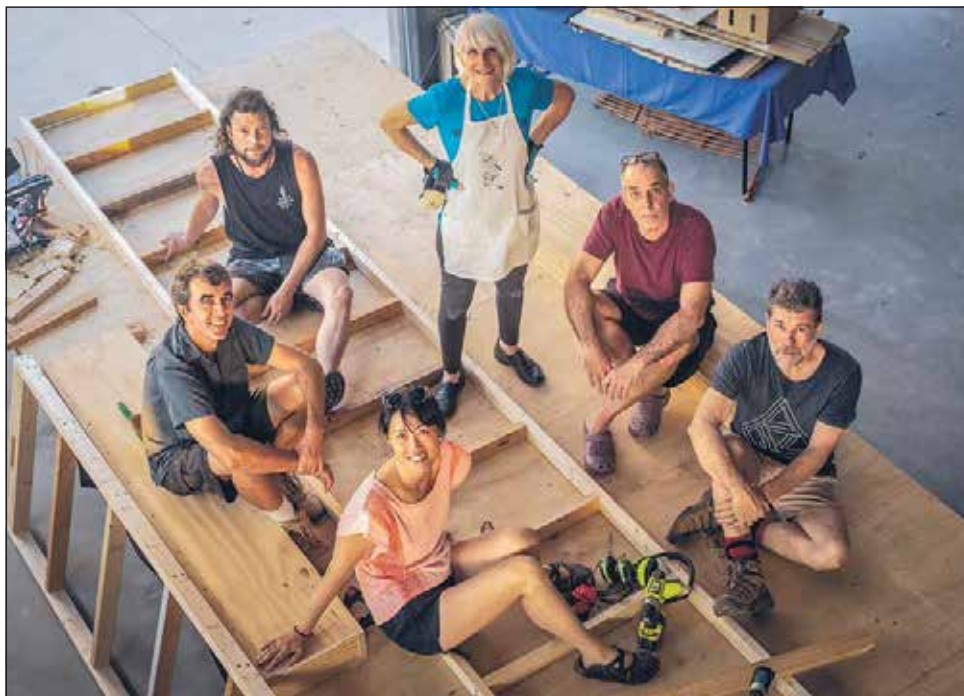
One Roof building crews Darren, Jacob, Patt, Duncan and Paul with Genevieve Lee (front) on the foundations of one of their new tiny homes. Photo Tree Faerie
