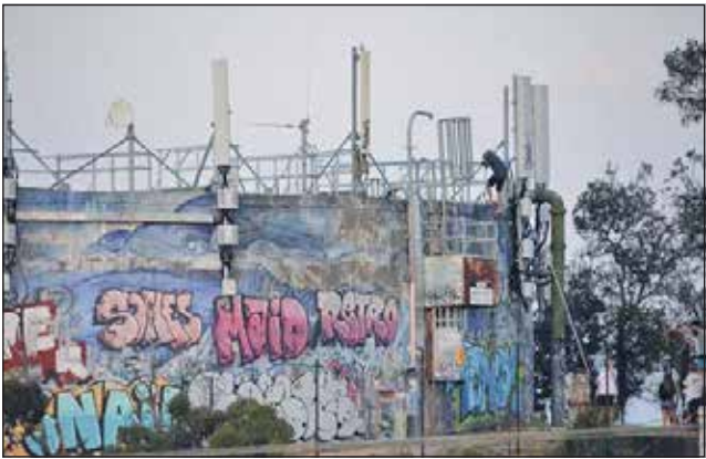
Paterson Street water reservoir. Photo www.imagesofbyronbay.com.au
