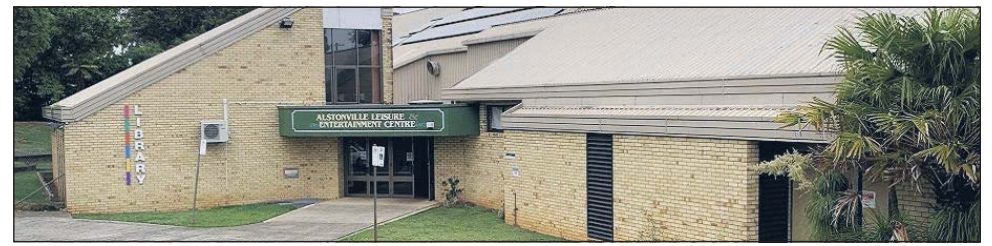
Alstonville's Leisure and Entertainment Centre is to become a film studio. Photo supplied
