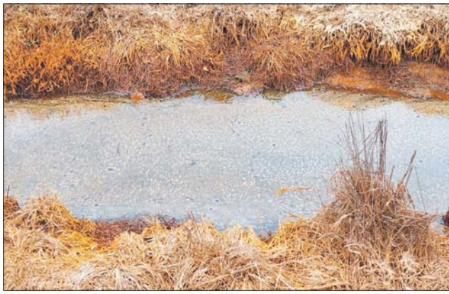
An environmental nightmare: drains full of soupy red water with nothing alive except mozzies, indicating acid sulfate soil. Photo supplied
