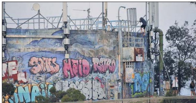
Byron's Paterson Street water tank.
