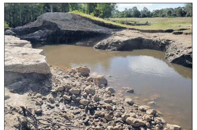
Flooding is so severe and stream speed during flooding so strong (up to 35km/h) that it has washed away part of the flood levee since it was repaired by Rous County Council. All three campsites proposed for the area are on the flooding side of the levee, as are toilets. Photo supplied
