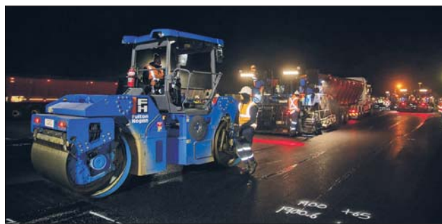
Airport resurfacing works. Photo David Lowe
