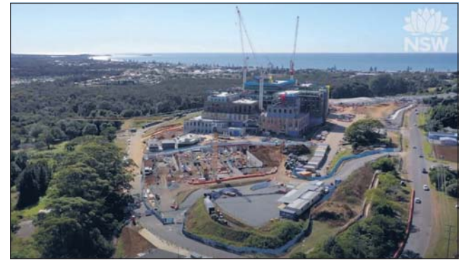
Tweed Valley Hospital construction. Photo supplied
