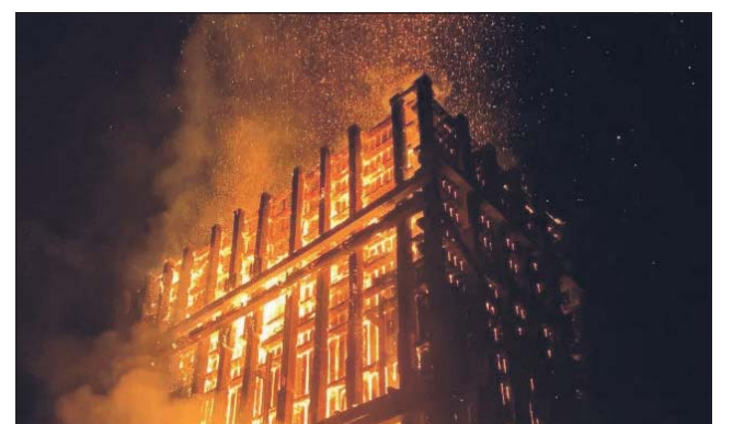
Fire has destroyed an old coal tower at Casino causing disruptions to the Brisbane-Sydney rail corridor. Photo supplied
