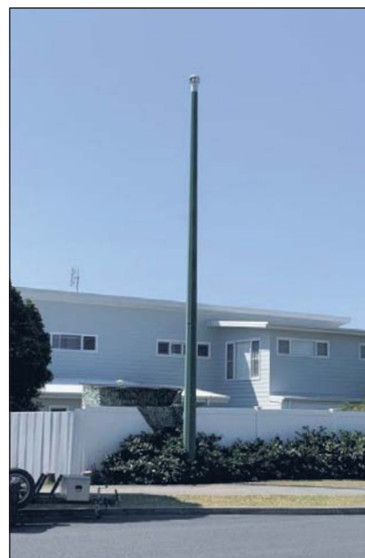
One of the vents at 1 Liriope Street, Casuarina. Photo supplied
