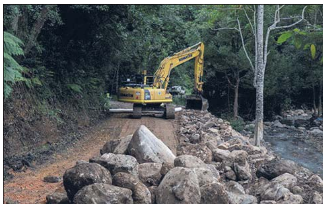
Palmwoods roadworks in Main Arm. Photo Byron Council
