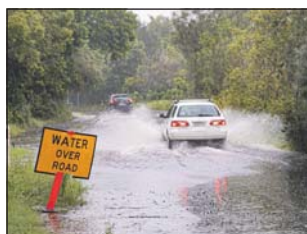
Council's 'water over road' sign has been in place for weeks - long before the recent flood event.
