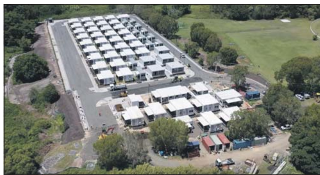
58 pods are located at 125 Tweed Street, behind the Brunswick Heads Sports Fields. Photo www.nsw.gov.au
