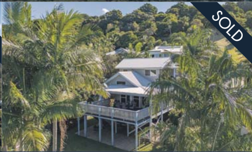
45 CORKWOOD CRESCENT, SUFFOLK PARK
