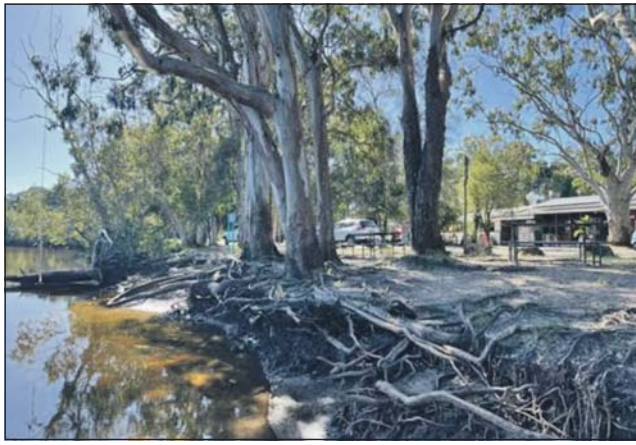
Marshalls Creek foreshore in New Brighton. Photo Byron Shire Council
