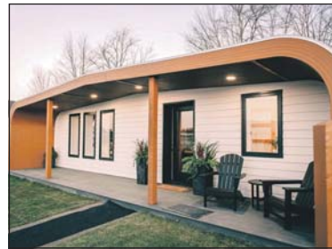
The BioHome3D is a proof-of-concept 3D printed house.
