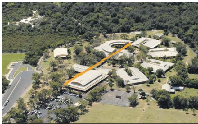
The Covered Outdoor Learning Area (COLA) proposal, as depicted by the Byron Bay High School's P&C. Photo supplied
