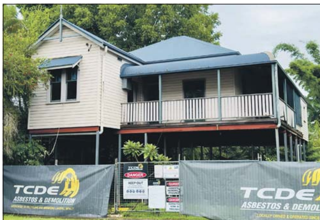
House scheduled for demolition at 29 Junction Street, Lismore. Photo supplied
