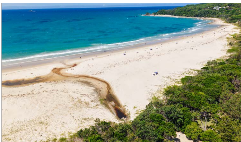
Drone shot of the Clarkes Beach stormwater outlet. Photo Jeff Dawson
