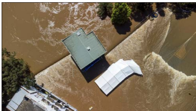
Floodwater surges over the levee at Browns Creek Pump Station, Lismore, 30 March 2022. Photo David Lowe
