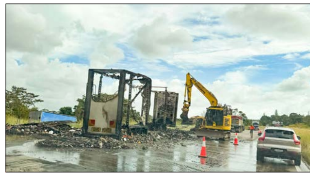
A truck caught fire on the M1 motorway at Knockrow, near Newrybar, last Thursday, resulting in big delays for those heading north. Photo supplied
