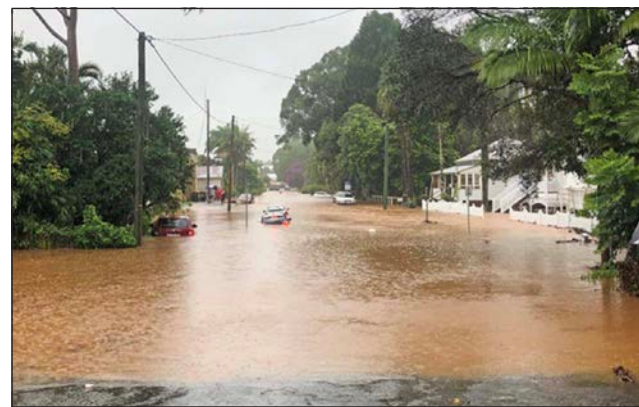
Flooding on Deacon Street, Bangalow in March 2022. Photo Byron Shire Council
