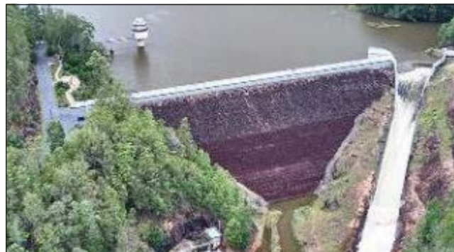
The existing dam wall at Clarrie Hall Dam. It is proposed to raise the wall by 8.5m to future-proof the Tweed's water supply. Photo supplied
