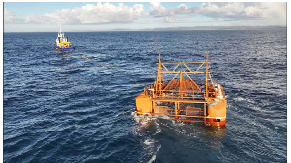
The 50-tonne artificial reef being towed into position to be sunk 3.5km off Patches Beach. Photo supplied
