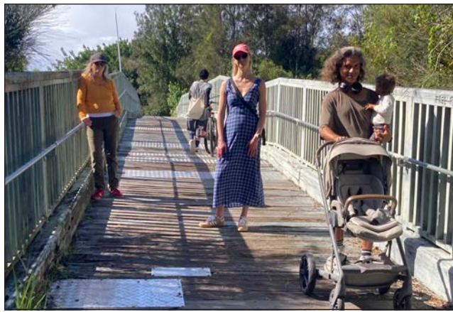
The Helen Street Bridge is a vital link for the local community. Photo supplied
