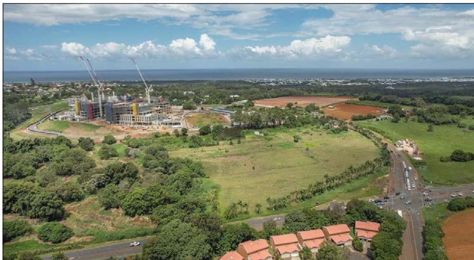
Tweed Valley Hospital during its construction. Photo supplied
