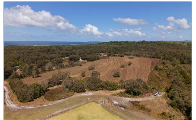
Clarence Property has slashed the site as they begin work on the frog retention ponds. Photo supplied
