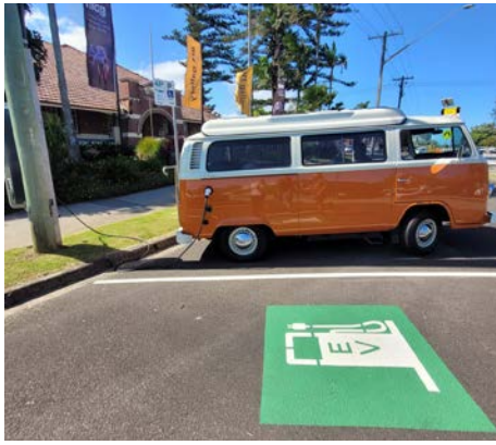
EV charger installed in the Ballina CBD. Photo Terry Teoh
