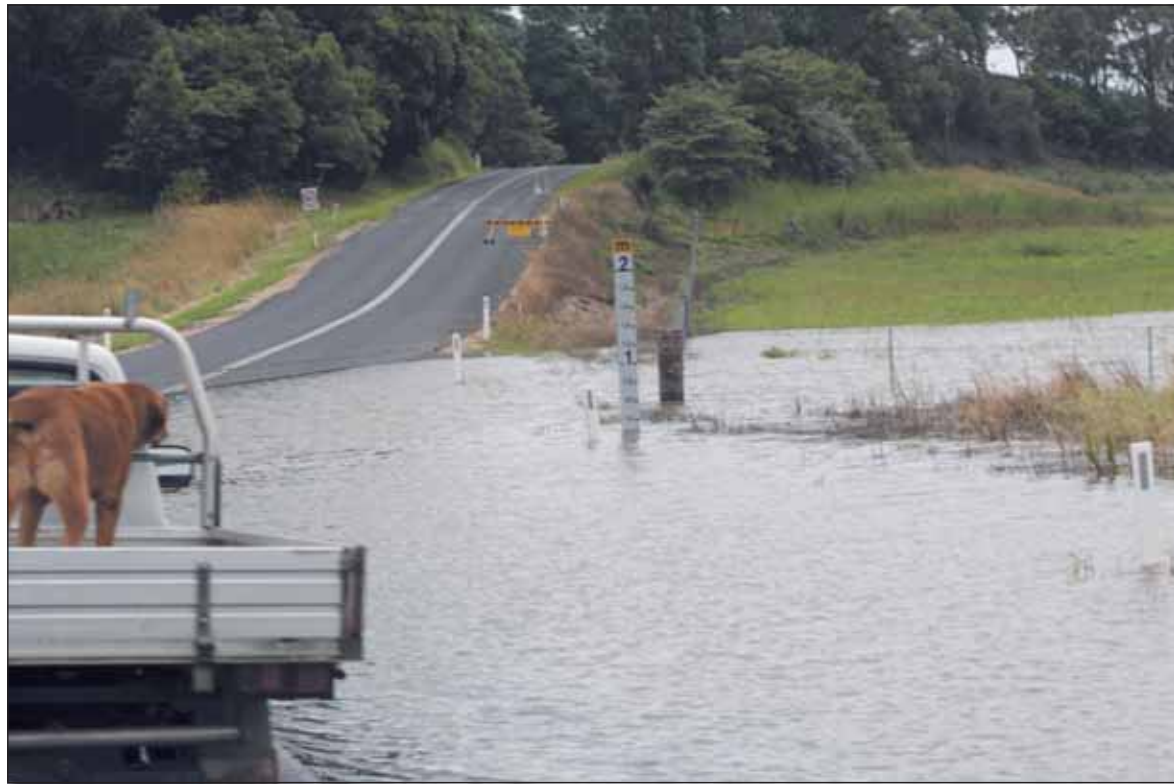
Wooyung Road was cut off to most traffic on Tuesday. Although there are worse floods to the north and south of Tweed Shire, the RTA advises people to make only essential journeys. Photo Jeff 'No Weather for Dogs' Dawson
